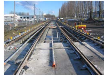
Stage 3: Concreting
