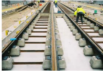
Stage 2: Track levelling
