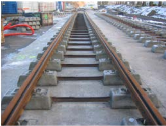
Stage 1: Sleeper & rail laying
